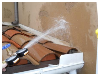
Water testing suspected area
