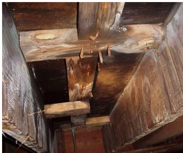
Subfloor damage due to leak
