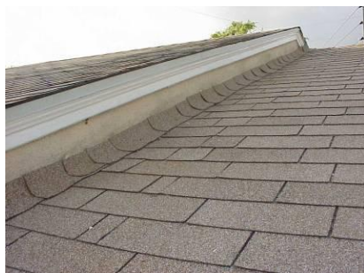
Roof with no proper counter flashing
