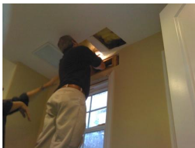
Cutting openings in ceiling
