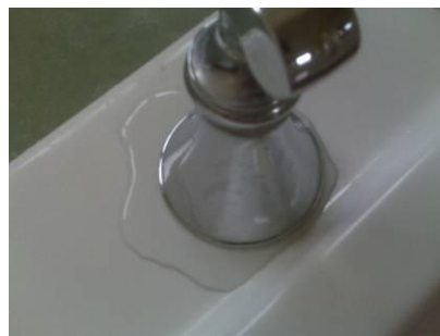
Plumbing fixture leak
