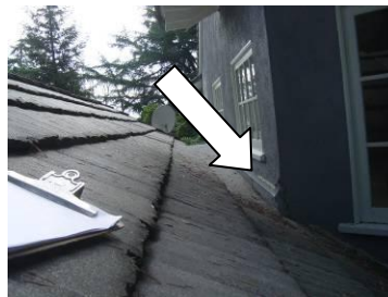
(D) Arrow showing point of water entry at flashing
