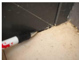
Openings at exterior lacking proper sealant
