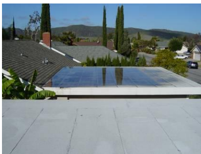
Roof not pitched properly to drain (holding water)
