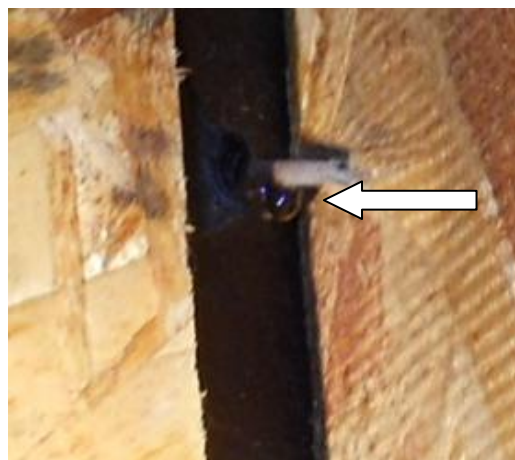
Close up of nail with drip
