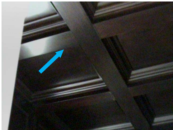
Figure 4. Thermal Imaging quickly identified the location of moisture; now it is up to us find the source of the leak.
