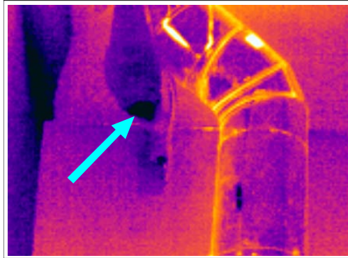
Figure 3. In the images above, water was condensing on and then dripping down from the refrigerant line down into cabinet. Thermal imaging helped map the leak to its source.
