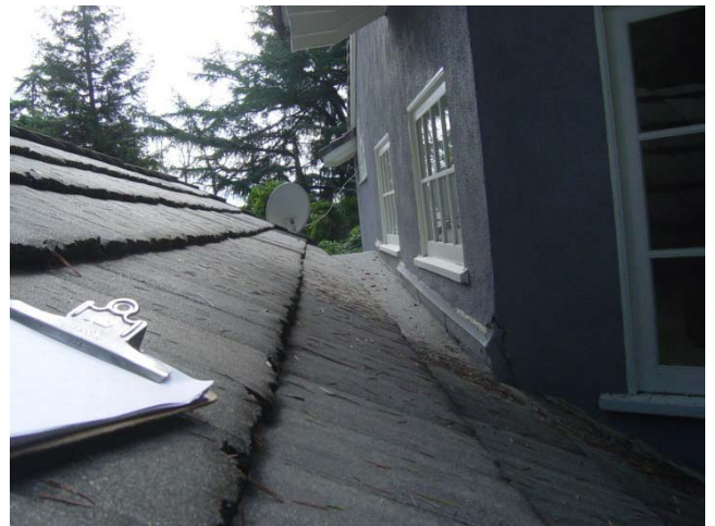
Figure 18. The wet area identified in thermal image was first confirmed with a moisture meter at 100% and then to the source. The roof had a steep slope with an upper roof cascading over, causing water to first hit the structure and bypass the counter flashing therefore leading to moisture entry. The suggested repair on this home involved a new design for a valley flashing versus the suggested roof replacement.
