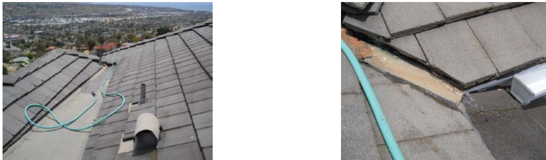
Figure 29. Our attention was now directed toward the roof with water testing. While on the roof and focusing our efforts on upper areas, we identified what appeared to be a new gutter system installation. When the contractor was questioned on this, it was determined that the gutters were installed just weeks before the initial water damage manifested.
