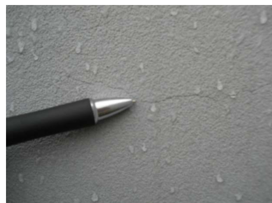
Figure 24. We now needed to locate the source of entry. Thermal imaging of the exterior of building quickly identified an anomaly which captured our attention. Upon closer look, we were able to confirm these anomalies were consistent with cracks in the stucco. As you can see in the photo on the right, the stucco finish was non-absorbent (acrylic finish). These cracks were actually breaks that allowed the point of entry. This collection of water and evaporative cooling are clearly shown in the thermal view. The fact that the finish of the stucco did not allow entry (except at crack) also meant it did not allow the trapped water to escape. Water simply took the path of least resistance and bypassed the window flashing to enter the building. Case solved!
