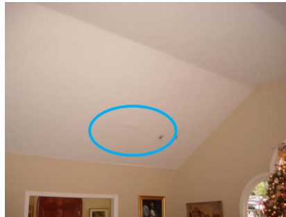
Figure 17. Left, visual image of leak (into blue bowl) centered in passage way between rooms. Center, visual image with circled possible water damage. Right, thermal image reveals wet area in ceiling. The arrow to lower left indicates how the water travels down the ceiling to the header wall directly over the catch basins.
