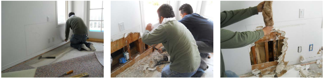
Figure 28. Destructive testing confirmed what the thermal imaging had indicated as drenched insulation above planter. Notice the worker wringing out water from insulation taken from wall.
