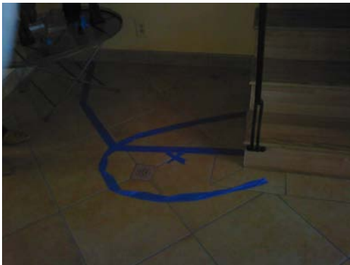
Figure 9. Through the use of thermal technology, we were able to map out a suspected leak location. As you can see in the picture on the right, the plumber is digging right at the "X".
