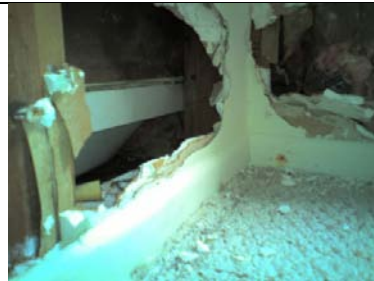
Figure 14. The wall was opened up to confirm the suspected leakage in the shower pan. Note: Dark area was wet at slab.
