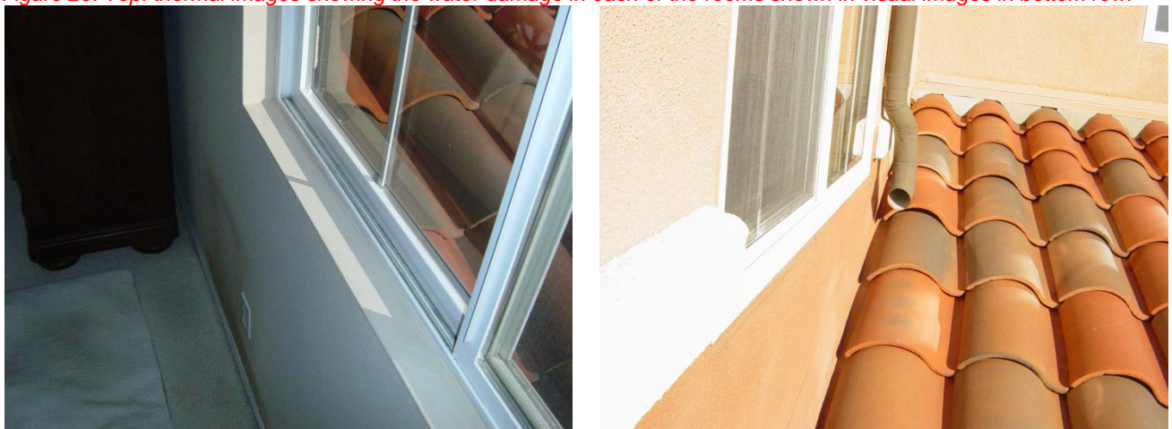
Figure 21. Upon review of the outside, it was found that the downspout from upper roof was directing a large amount of water against the side of the structure, bypassing the counter flashing and leading to water entry.
