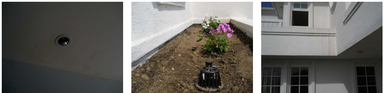
Figure 26. The living room of this large custom home showed a leak at the ceiling corresponds to a planter on the exterior of the building as seen in the center image. The right image is the outside view that corresponds to the thermal image in Figure 25 of the gentleman taking a moisture reading. The contractor completely removed and re-waterproofed the planter, believing the moisture was a direct result of the proximity of the planter. The ceilings of living room and adjacent room were all repaired. However, with the next rain, the same leak reappeared.
