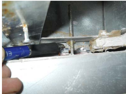
Figure 23. The frustrated builder had cut many holes in the walls in an effort to find the leak (left photo). Through our efforts, we were able to duplicate the leak, and as seen in the photo on right, determine the leakage just under window flashing.
