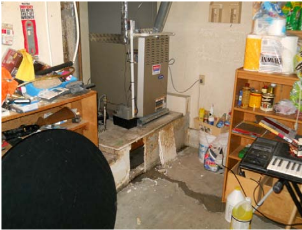
Figure 7. A definite leak is shown at garage floor. The opposite area in lower hallway showed no sign of leakage or damage anywhere.
