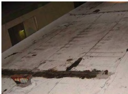
Figure 4. Visual of substandard roof patch Figure 4a. Thermal image of substandard roof patch.
